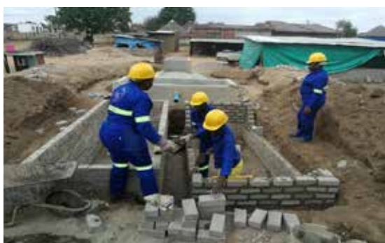
Image 21: Trainees finalising the construction of the compost pits for a 12 cubic metre digester constructed at Manjonjo Farm in Magoro.
