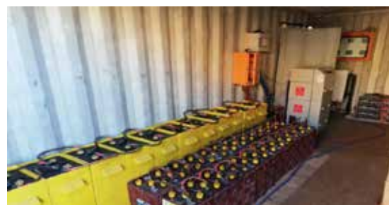
Image 15: Auxiliary storage with lithium ion and lead acid combination batteries. The lead acid battery is on Powerstar2 and the lithium ion is on Powerstar3/Nomad.
