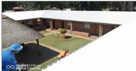
Image 6: SANEDI personnel at the newly Cool Roof painted residential blocks of the SANDF legacy project at Sekutupu Old Age Home opened by the Minister of Defence.
